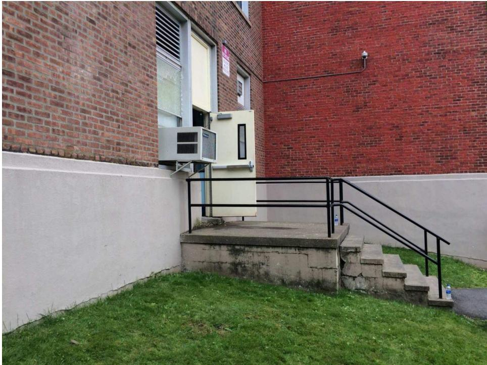
Category 70: Exterior Stairs, Steps, and Ramp Foundation at rear stair is in disrepair. Repointing and masonry replacement required for auditorium exterior entry stair.
