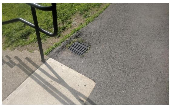
Category 46: Catch Basins/ Drop Inlets/ Manholes Install drainage along driveway in front of school to eliminate icing/ponding and erosion. Replace yard drain at stair in playground area with larger structure and piping to eliminate icing/ponding hazard and erosion.
